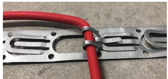
5. Place thumb on the secured cable and bend the cable in the direction of the next loop
