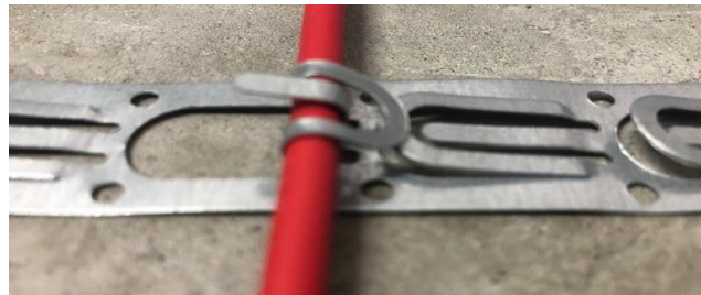
3. Fold the loop all the way over the cable and the "middle finger"
