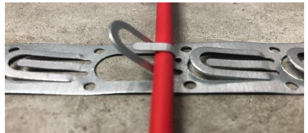
2. Place the cable in the V and fold the "middle finger" over the cable
